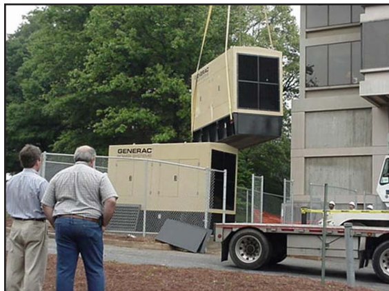
MPS gensets are smaller and easier to transport than huge, single engine generators.
