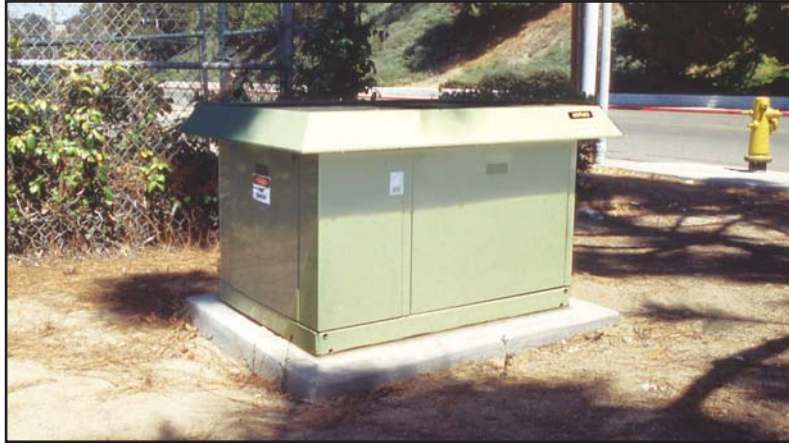
Cox's Generac gensets ensure high service reliability throughout its network.
