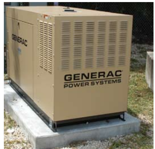
25 kW QT Series propane fueled gensets
