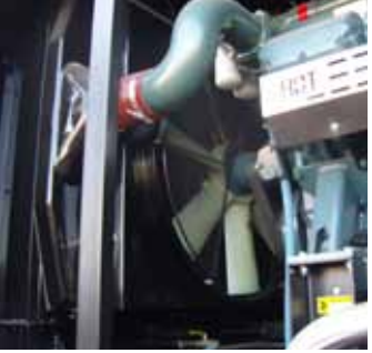
The Generac Bi-Fuel Gemini MPS systems are poised to kick into gear in the event of a power outage. The three units installed operate in parallel to provide consistent and reliable backup power.
