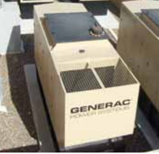
The Generac Bi-Fuel Gemini MPS systems are poised to kick into gear in the event of a power outage. The three units installed operate in parallel to provide consistent and reliable backup power.
