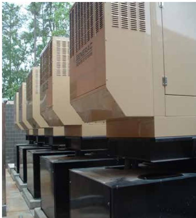
generators start up and parallel in a matter of seconds, without switchgear. With the paralleling capability and redundancy built into its system, Generac's modular approach really made sense for our project."
