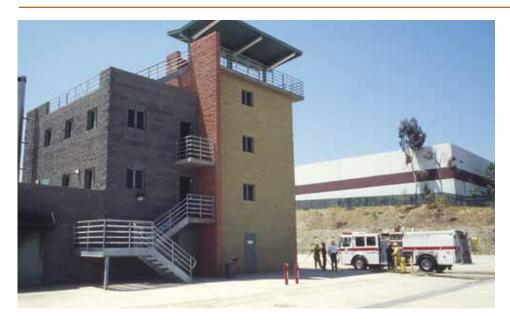
training, a burn room for real fire fighting practice, and walls for climbing or rappelling," Bales explains. "There are stairs with balconies at different elevations and wooden props for smoke ventilation practice. The water pumping system uses recycled well water and can be used for hose tests and fire engine pump testing. The tower also has facilities for practicing hose lays and ladder drills."
