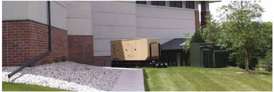
Installed in March of 2002, the standby generator allows West Wood members to finish their workout, change clothes, and exit safely during a power outage. When running, the generator supplies power to the first and second floor, the hot water pump, elevators, and 104 emergency lights. The genset is equipped with a 300 gallon tank, and can run anywhere from six to seventeen hours depending on the electrical load it supports and the fuel available.
