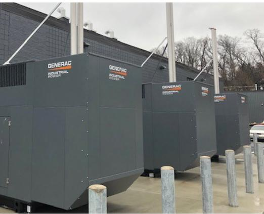
Roach said when considering a backup power solution, they really wanted redundancy and natural gas fuel. “We have natural gas available on site and using it instead of diesel reduced labor for us and makes everything more turnkey. We didn’t want to have to worry about diesel deliveries and tracking levels.”
