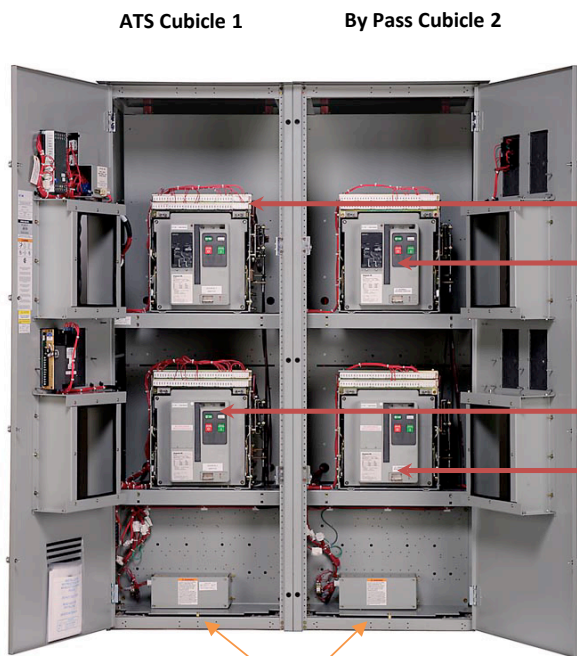
Multi Tap Transformer
