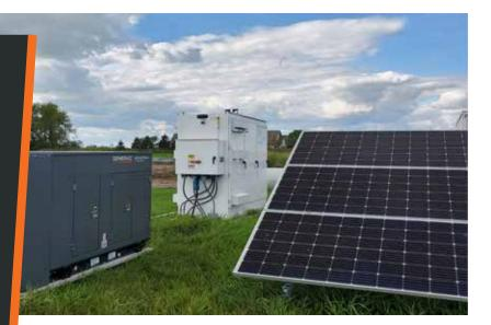
"The generators are used to charge the batteries on days when the sun is not shining, and the batteries have been depleted. This adds a level of resiliency to the system and guarantees it will always be operational."
