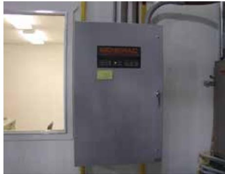
load transfer to occur in this manner, without delay. The design of the CTTS makes possible the voltage synchronization between the utility and the running genset prior to the transfer, and allows the load to be safely and quickly shifted from one source to the other without delay or dangerous backfeed.
